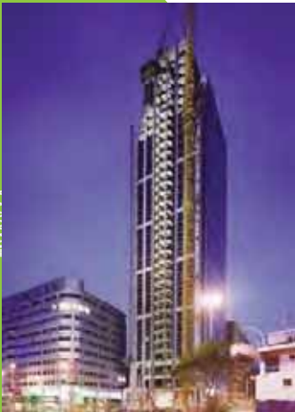
BubbleDeck's height saving allowed 2 floors to be added during construction
